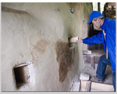
Figure 6.16d How wood would be stoked into a chamber of the noborigama kiln at the Shigaraki Ceramic Cultural Park, Japan (photograph by Carol Ventura, 2006).
